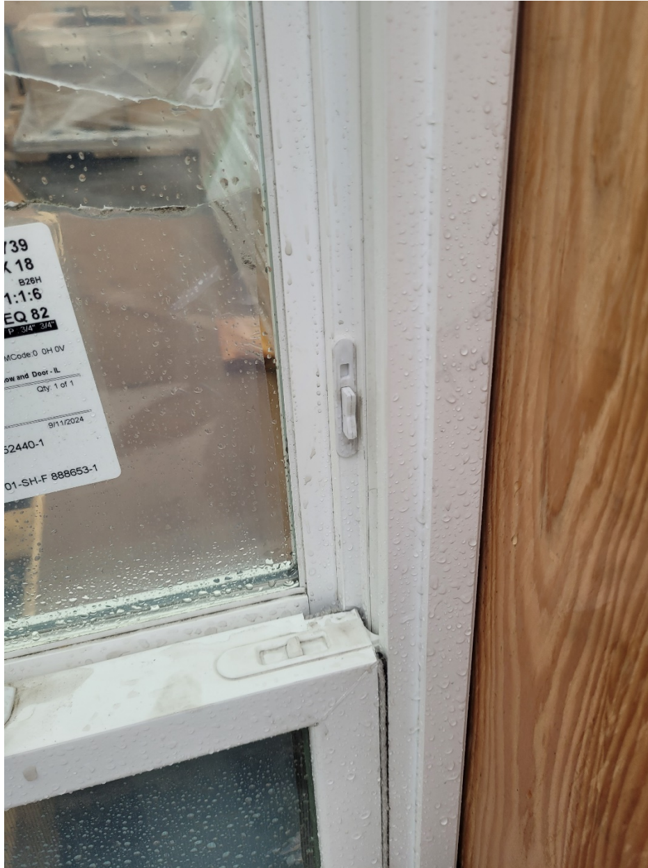
Photo 1 WOCD installed into frame
